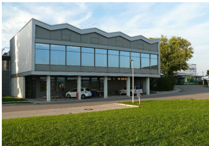
Front view of the lecture hall
